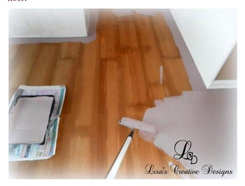
Apply two coats of primer to the floor, letting each coat dry in between applications.
