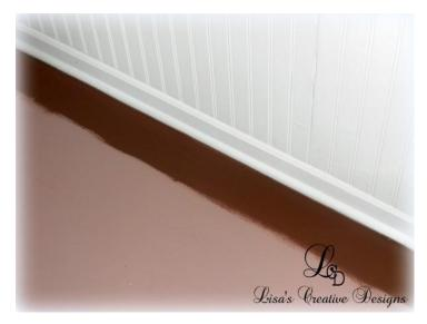
Apply two to three coats of the Porch and Floor Paint with a roller, waiting for each coat to dry in between. Let the floor dry overnight.
